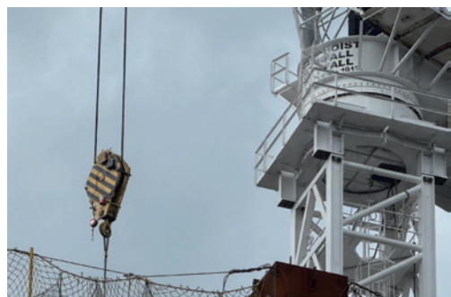
Construction Site Operation
