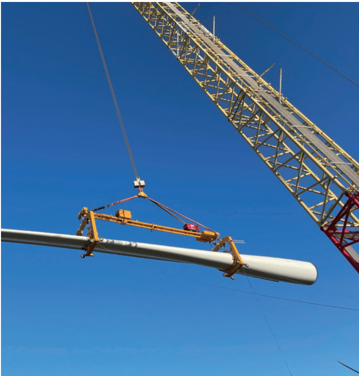
Wind Turbine Installation
