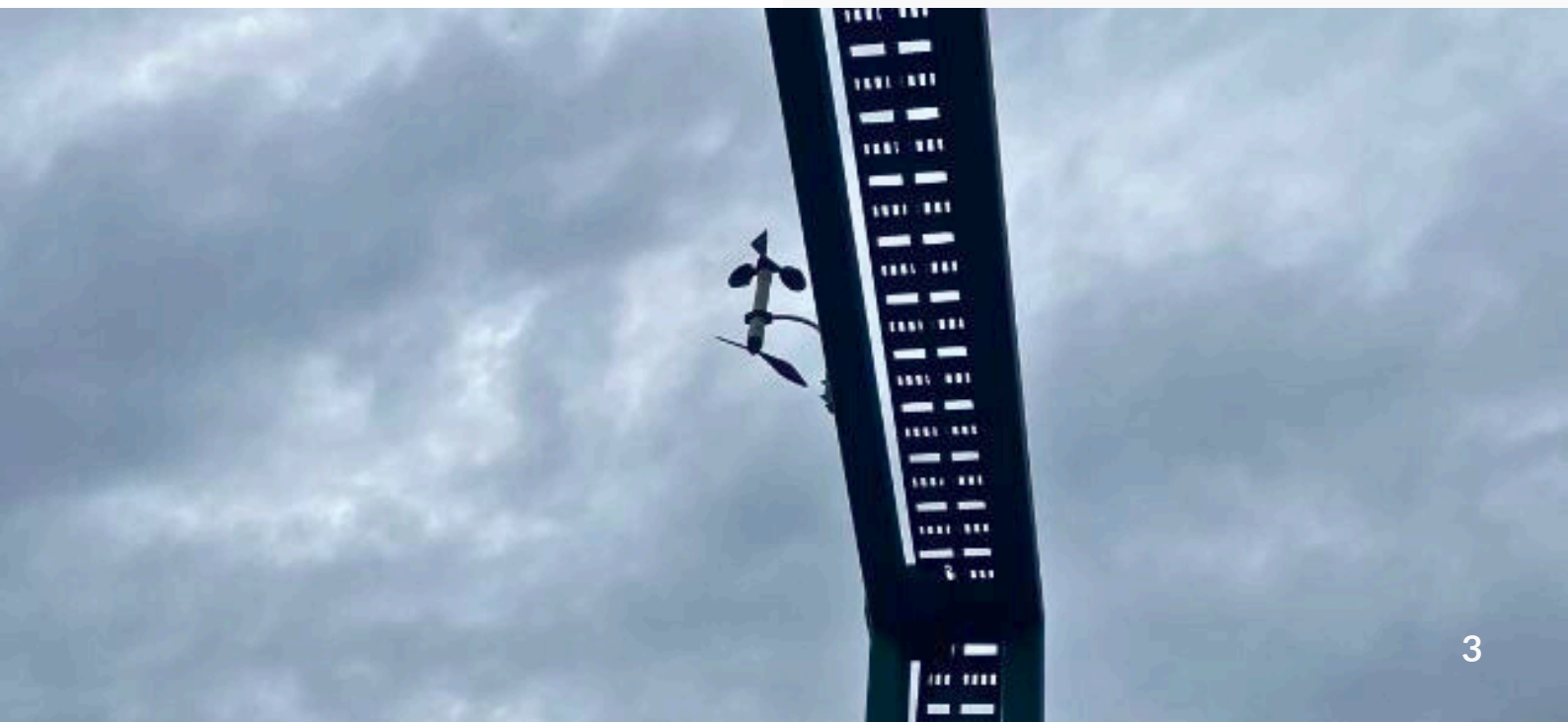
▼ WindPro wind sensor installed in empty container yards
